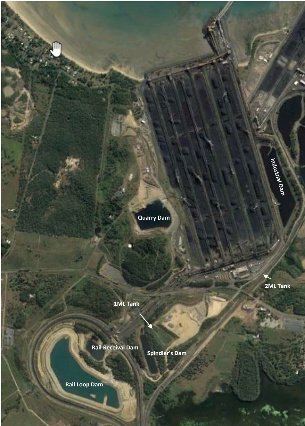
Figure 6: Water Management Infrastructure
