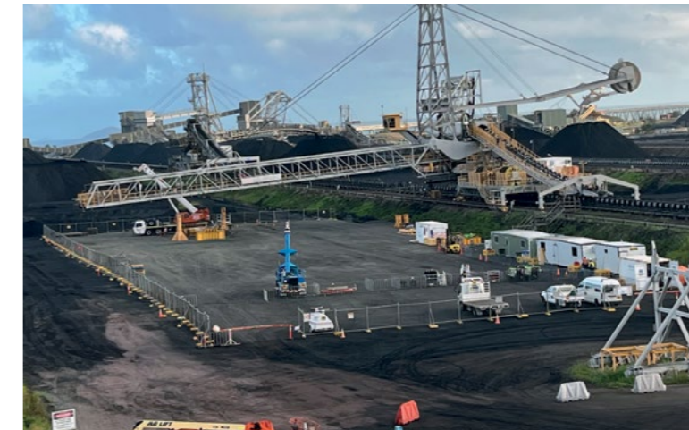
Figure 15: ST1 deconstruction before and after
